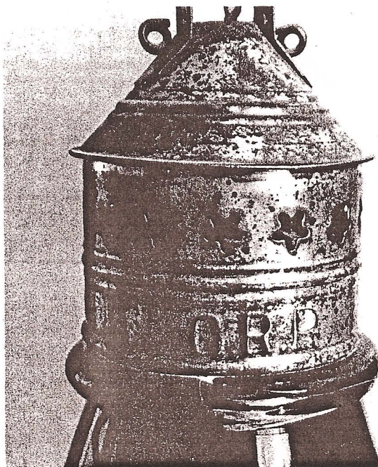
Figures 3.39 and 3.40 - This "Star pattern" lantern (STP-3) is stamped "C.R.R." (Concord Railroad) on the side of the smoke dome. The red flashed globe is unmarked. Collection of Tom Stranko
